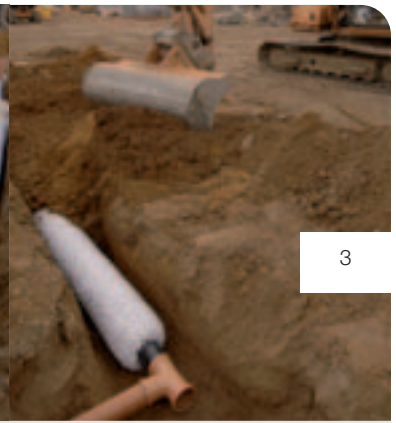
Arisings used to backfill to top of trench.
