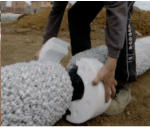
Ezy-Drain sections are simply joined together using standard 110mm fittings and junctions. Joints may be protected with the optional polystyrene collars or simply backfilled with as-dug material.
