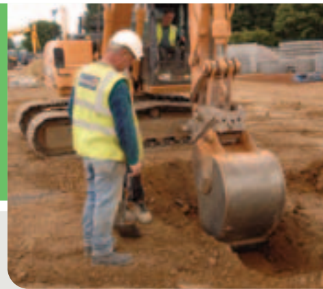
Trench excavated to site specific requirements arisings kept for re-use.
