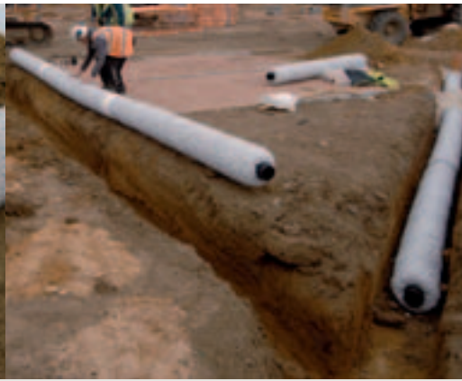
Assembled Ezy-Drain system is then rolled into the dug trench.
